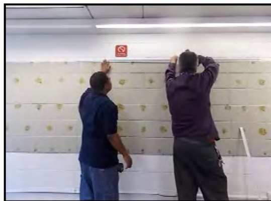
Dry erase board installation in progress.
