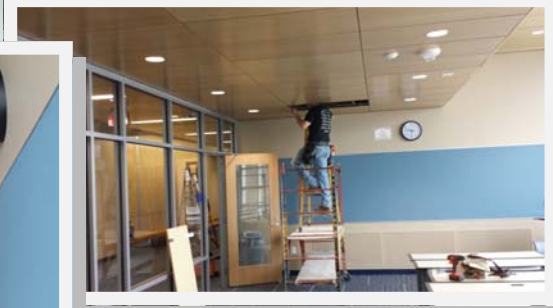
Installation of ceiling retaining clips
