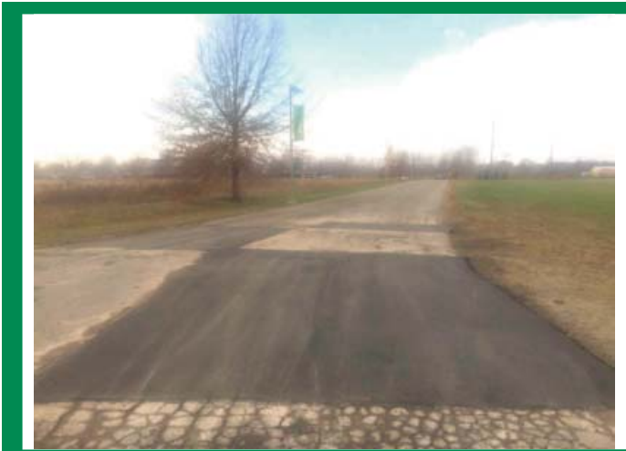
Emergency asphalt repairs at the Western Campus
