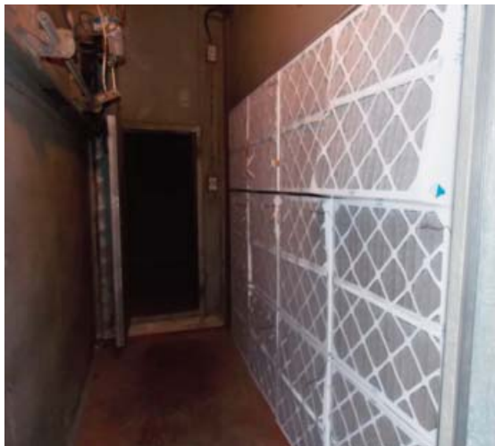
Preventive Maintenance of the building mechanical systems: Maintenance staff has changed the pre-filters and the bag filters on main air handling units.
