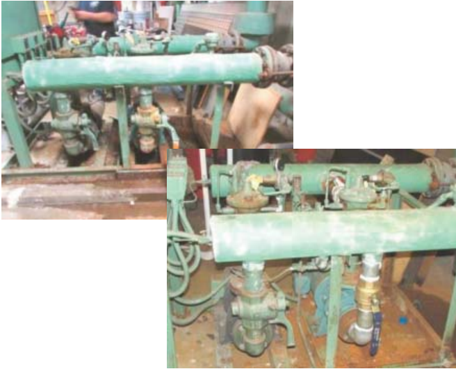
Preventive maintenance of the building mechanical systems. Inspection and replacement of the District Office water system pump.
