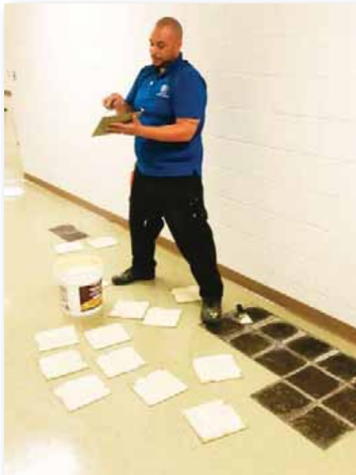
General Maintenance Repairs at the Northwest Campus
