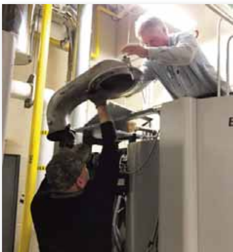
Northwest Campus Boiler Inspection and Repairs
