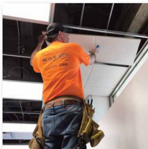
Northwest Campus Police Authority Renovations
