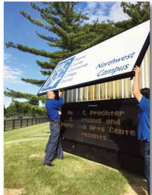
Northwest Campus Marquee Repairs
