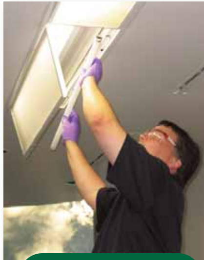
Downriver Campus Lighting Repairs
