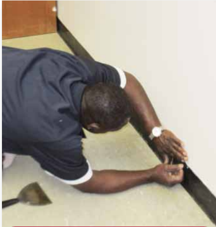
Downriver Campus Drywall Repairs
