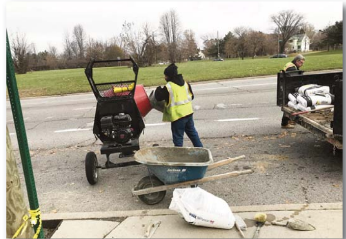
Eastern Campus Cement Repair Project
