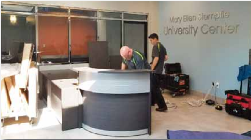
Mary Ellen Stempfle University Center Lobby Renovations
