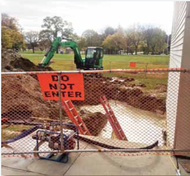
Northwest Campus Waterproofing
