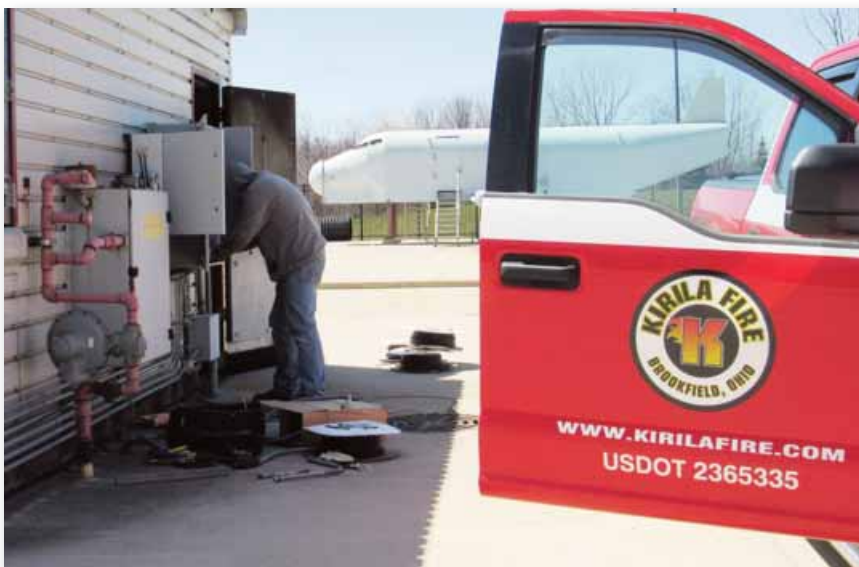
Downriver Campus Kirila Fire Repairs to Burn Room
