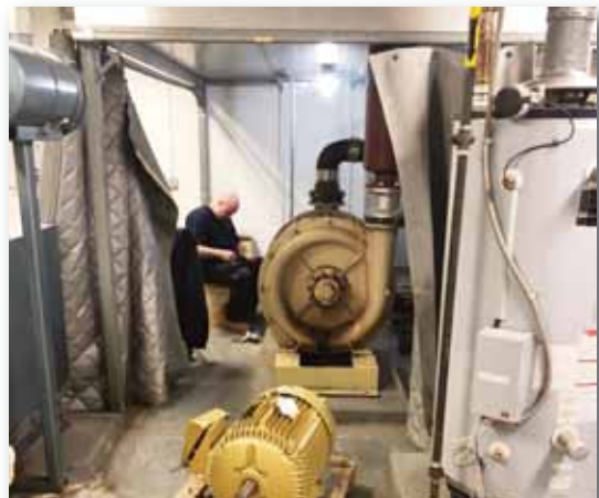
Northwest Campus Equipment Inspection and Repairs
