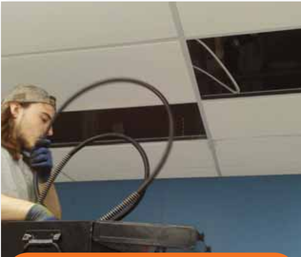
Downtown Campus Water Valve Ceiling Repairs
