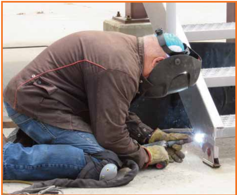
Downriver Campus Welding Repairs
