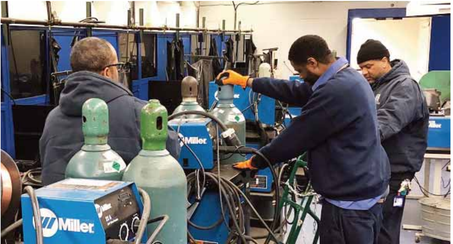
Preparing the Welding Lab for the First Day of Classes
