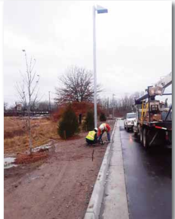
Ted Scott Campus Light Pole Installation
