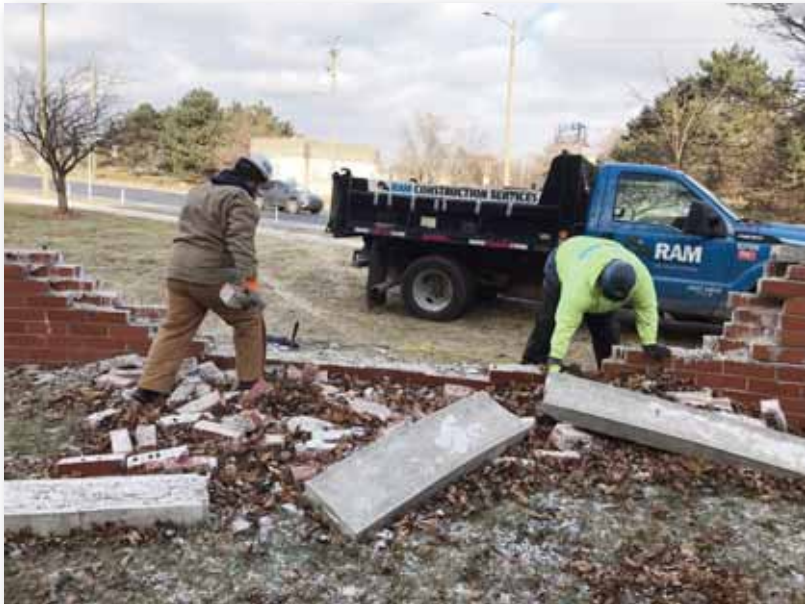
Eastern Campus Screen Wall Repair
