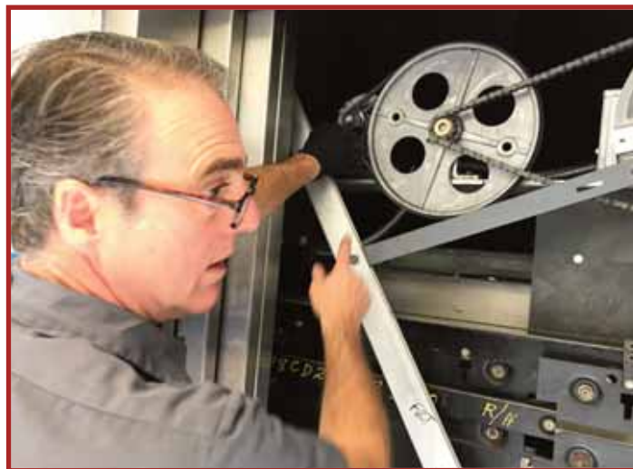
Eastern Campus Elevator Inspection
