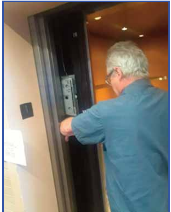
Elevator Equipment Repairs Ted Scott Campus
