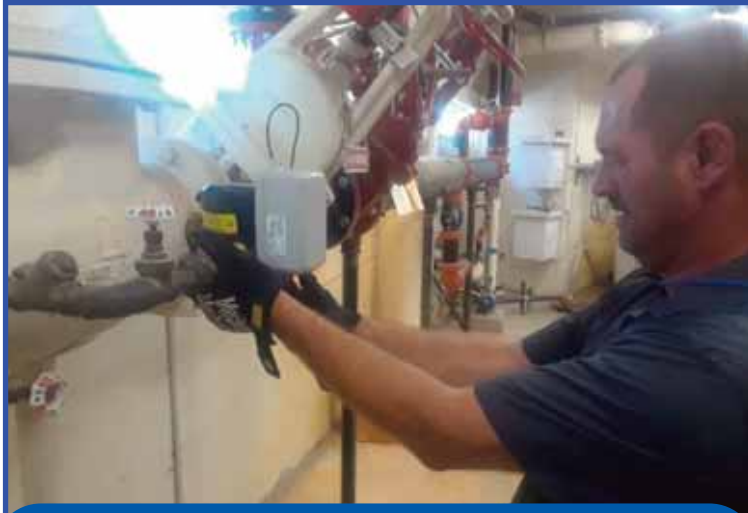
Fire Protection Meter Installation Ted Scott Campus
