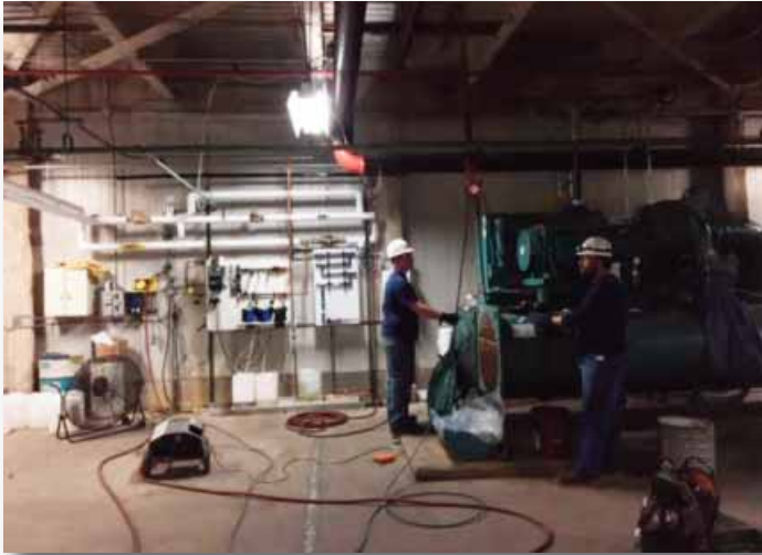
Johnson Controls visited the Curtis L. Ivery District Office Building to flush and clean the air conditioning system.
