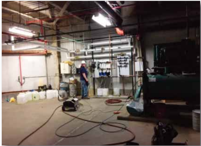
Johnson Controls visited the Curtis L. Ivery District Office Building to flush and clean the air conditioning system.
