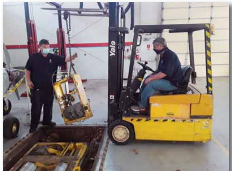
Downriver Campus/Auto Bay Dynamometer Removal to Enlarge Instruction Area.
