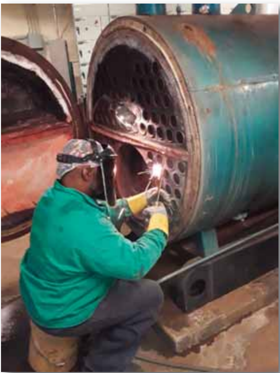
Ted Scott Campus/Boiler Tube Welding
