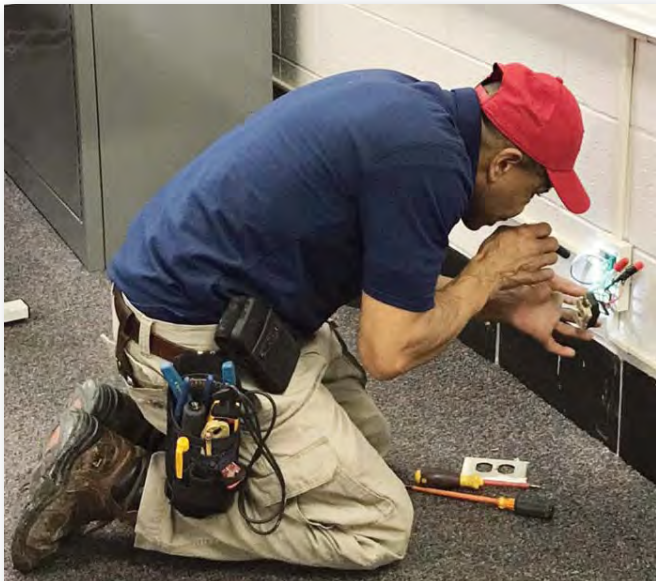
Eastern Campus Fashion Design Lab Equipment Installation
