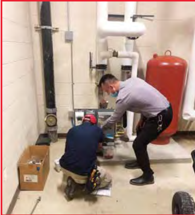
Booster Pump Repair
