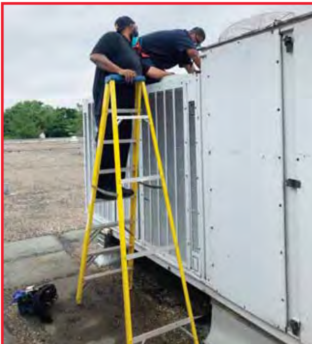
HSC Building Repair
