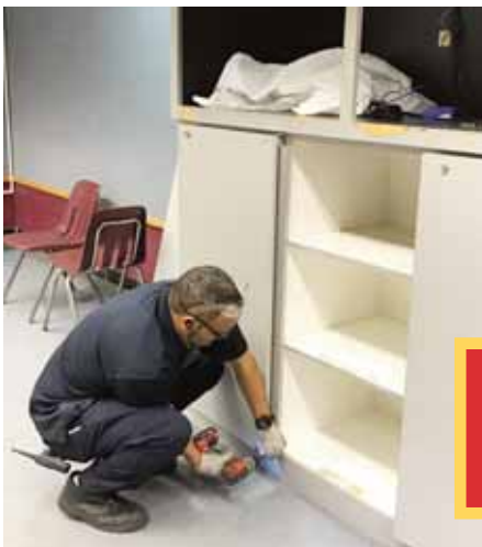
Eastern Campus ITV Cabinet Dismantle Project
