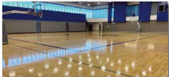
A vendor specializing in the maintenance of athletic wood flooring and facilities applied a new high gloss Protective finish to the 15,000 square foot floor of the Thomas E. Howard Junior Arena.
