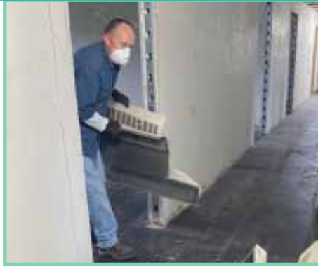
Plumbing/Heating Demolition within the AAB for the Detroit Police Academy Renovation
