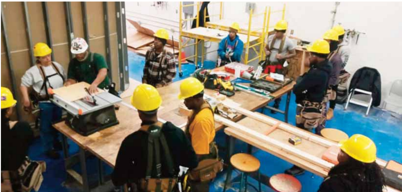
Students in the Construction Trades Training Program are learning to layout floor joists.
