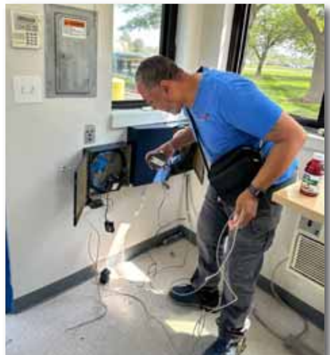
Data line repair in Security booth.
